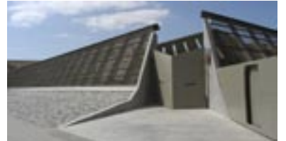
17 INFANT WING OF NESTOR ALAMO STATE SCHOOL Architects: Manuel J. Feo Ojeda, Juan J. Espino Duran Completed: 2003 Address: Rambla de Jinamar, Las Palmas de Gran Canaria
