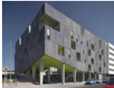
23 INAKASA BUILDING Architects: Alexis López Acosta - Xavier Iván Díaz Martín Completed: 2005 Address: Calle Harld Flick 8, Las Palmas de Gran Canaria
