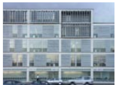
20 ADMINISTRATIVE BUILDING Architects: José Antonio Sosa Díaz-Saavedra, María Jesús González González Completed: 2005 Address: Avenida Alcalde Díaz-Saavedra Navaro
