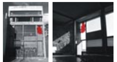
19 CASA RUIZ Architects: Magüí González Completed: 2005 Address: San Cristobal, Las Palmas de Gran Canaria
